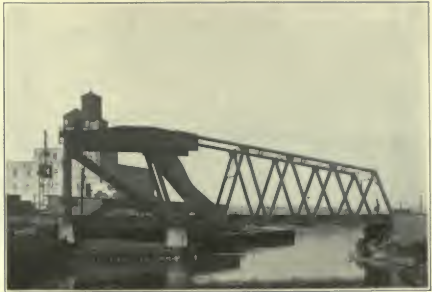
FIG. 264. BRIDGES. Bascule bridge of the Illinois Central Railroad, the Atchison, Topeka & Santa Fe Railway, and the Chicago & Alton Railroad, over the Chicago River at 31st Street and Archer Avenue.
